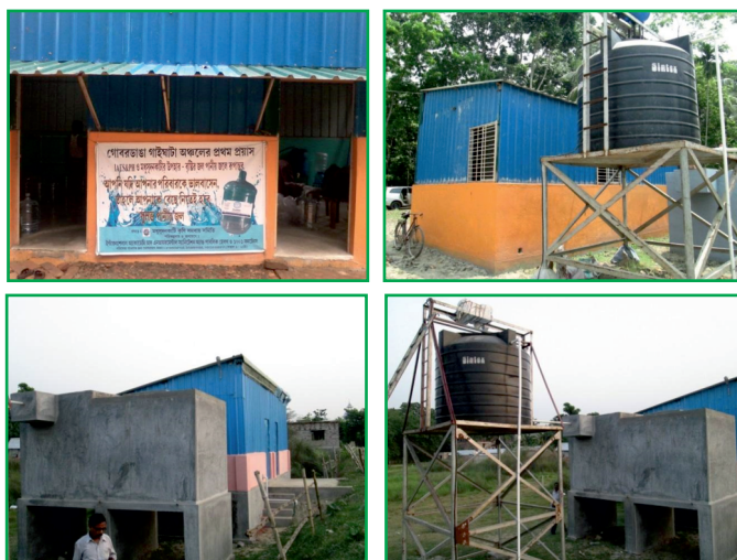
Figure 2. Purified Water ATM Plant at West Bengal
