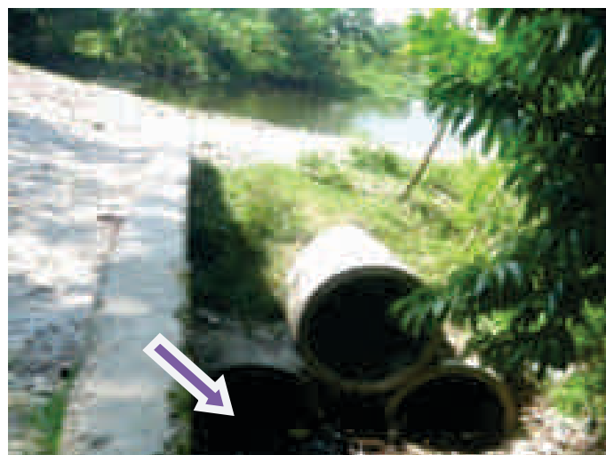
Figure 6: Solid waste accumulation at sewer outfall on the Mayur river, Chhoto Boyra (Shashan Ghat).
