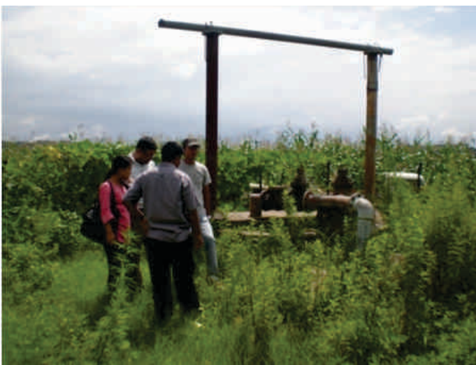
Figure7 : Newly Constructed Sump Well
