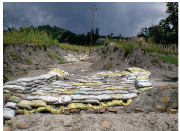
Figure 10 : Damage of agricultural land due to sediment flow from the sand mining site
